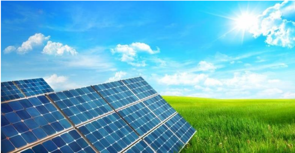
Solar photo voltaic system-with Net meter
